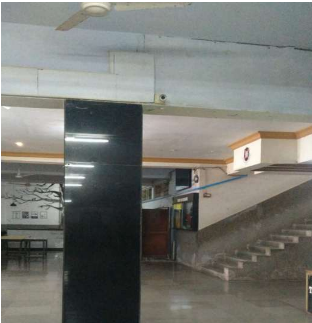
CCTV Camera in the Corridor
